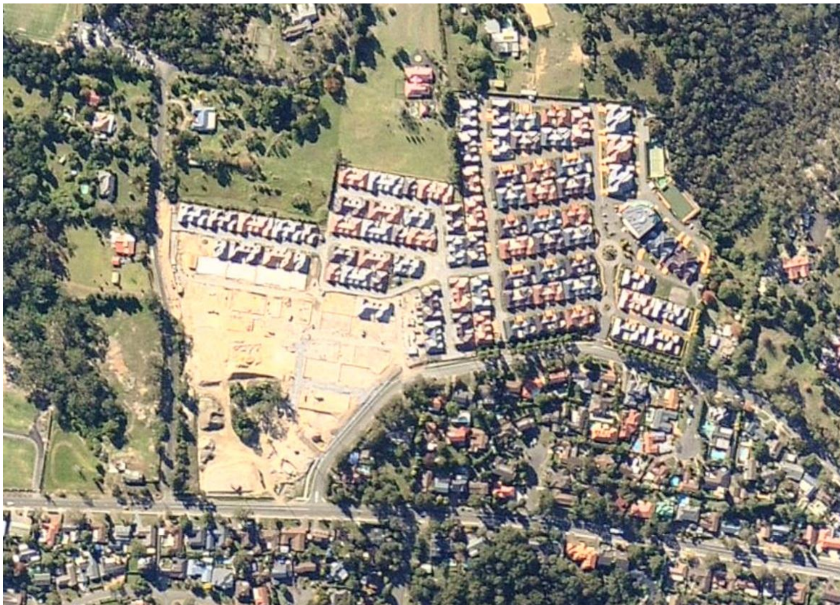
Figure 1 – Aerial Photo of Site (15 Old Glenhaven Road, Glenhaven) Source – www.nearmap.com/photomaps
